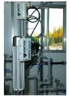
Kinitics deployed prototype actuators onto the wellsite with the intention of validating the core technology and discovering operational requirements. Two actuators were installed to operate the water and condensate dump valves, while a third would operate the backpressure control valve. It was quickly discovered that the smaller actuators did not actuate quickly enough for dump valve operation. The backpressure control valve actuator remained in operation for the duration of the test period.
